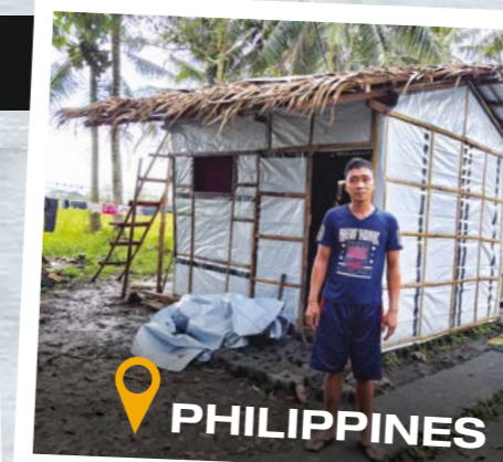
Following Cyclone Trami, people needed to construct temporary shelters before the next storm arrived. Here, the tarpaulins are held in place by batons over a bamboo frame and used to make the roof watertight, under a layer of palm leaves.
